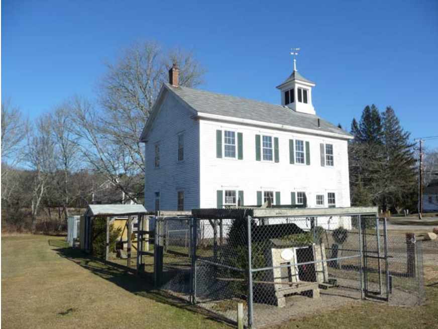
View looking southeast at north and west elevations.
