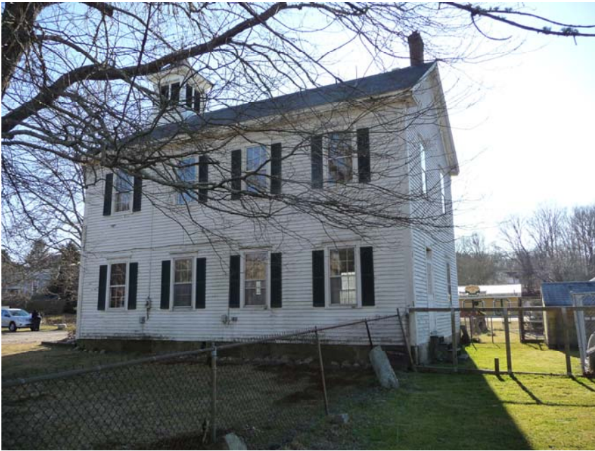
View looking west at east elevation.
