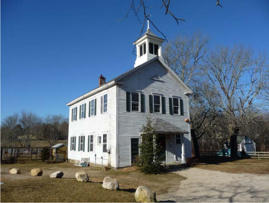
View looking northeast at façade and west elevation.
