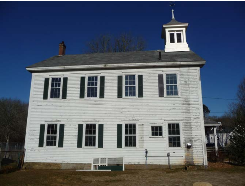
View east of west elevation.
