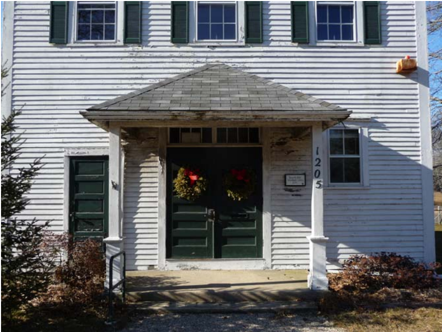
View looking north at entry.
