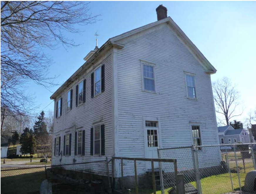
View looking southwest at north and east elevations.
