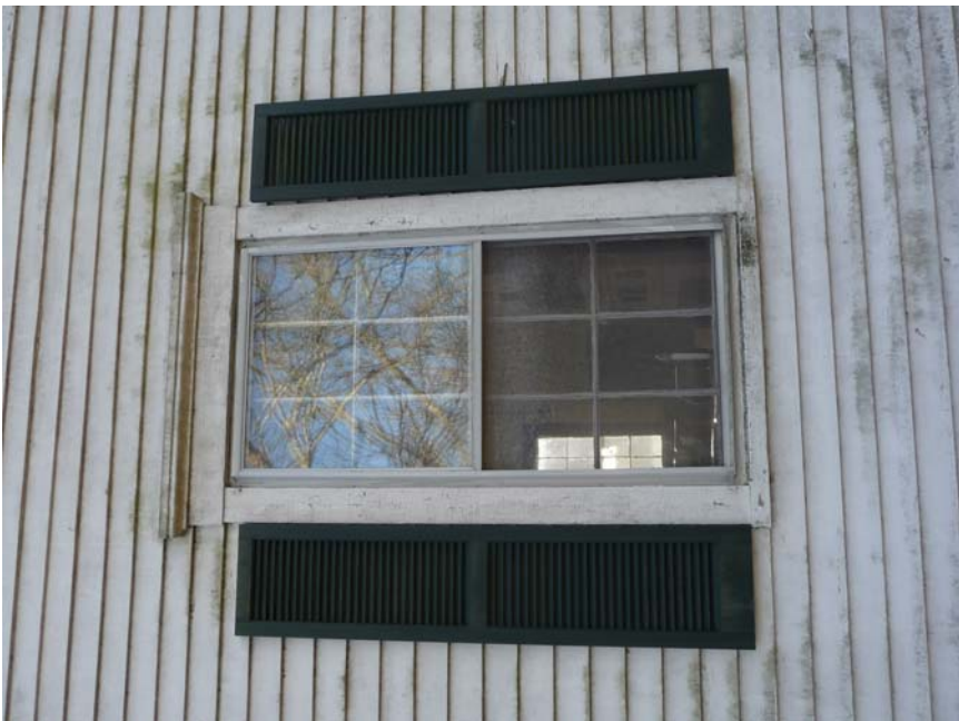
View looking west at typical window on east elevation.
