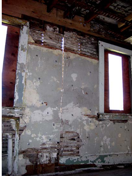
Figure 3. Interior view, kitchen wall, Elihu Akin House, 2008 (photograph by the author)
