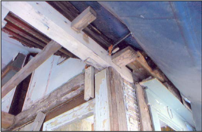
Rotted Top Plate Repaired
