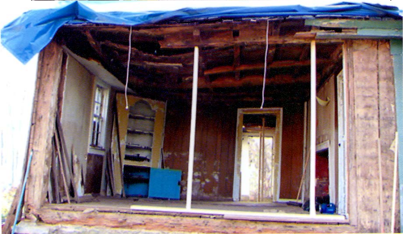
Rotted Top Plate Repaired
