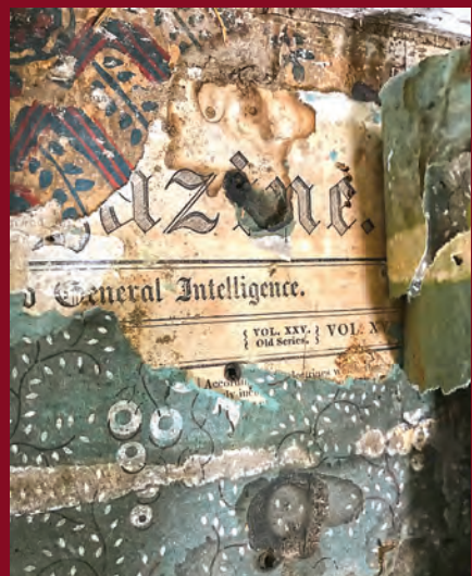
RIGHT Newsprint served as a base for applying a newer vine-patterned wallpaper in the mid-1800s.
