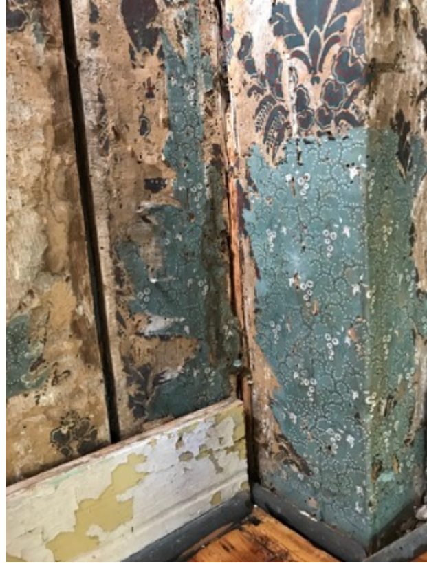
After surface cleaning
