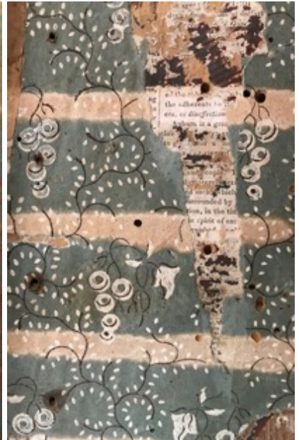
Fading of color due to contact with highly alkaline plaster
