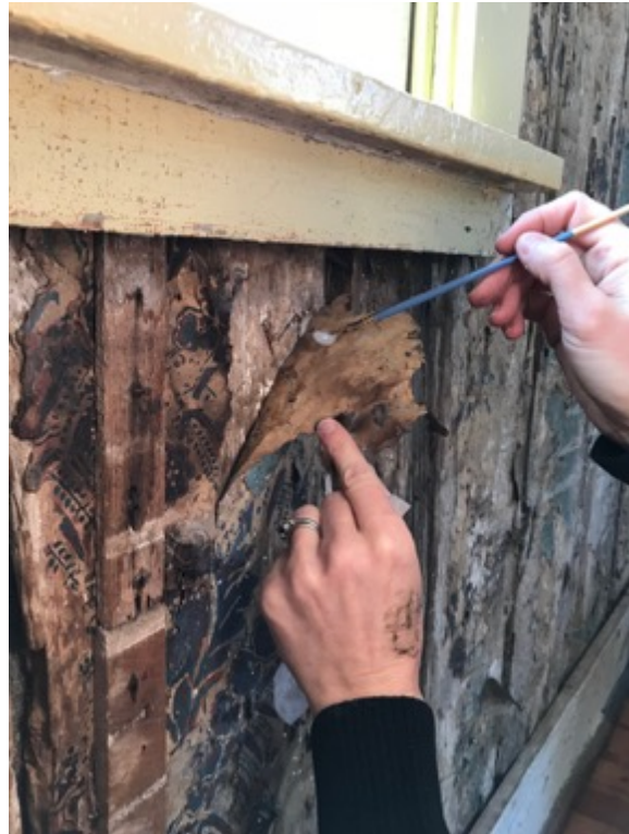
Detail of setting down with wheat starch paste
