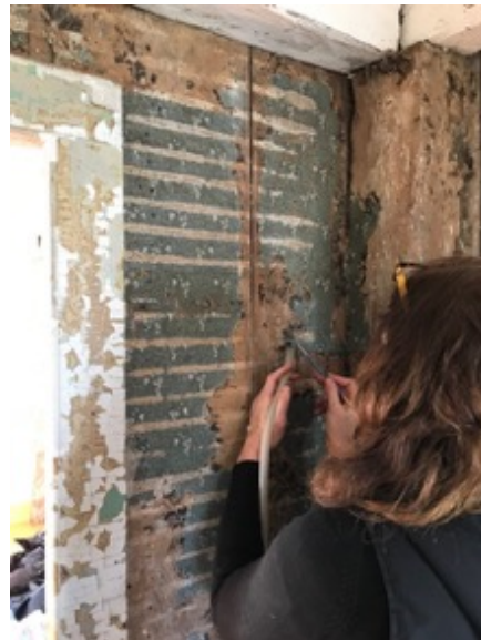
Removal of loose dust, construction debris and insect frass with a HEPA filtered variable suction vacuum
