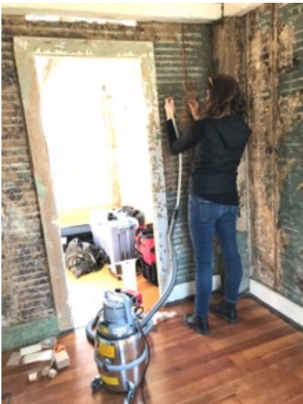
Removal of loose dust, construction debris and insect frass with a HEPA filtered variable suction vacuum
