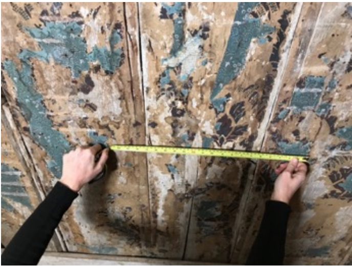
Measuring the roll width from seam to seam (south wall)
