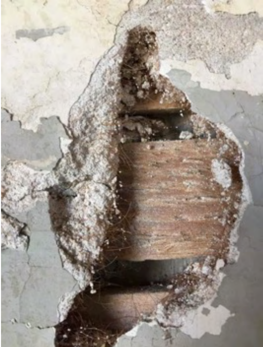
Underlying plaster & lath wall structure
