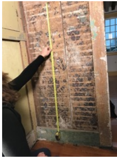
Measuring continuous paper height (east wall)
