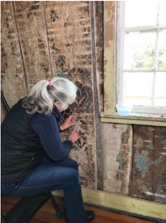
Setting down with wheat starch paste
