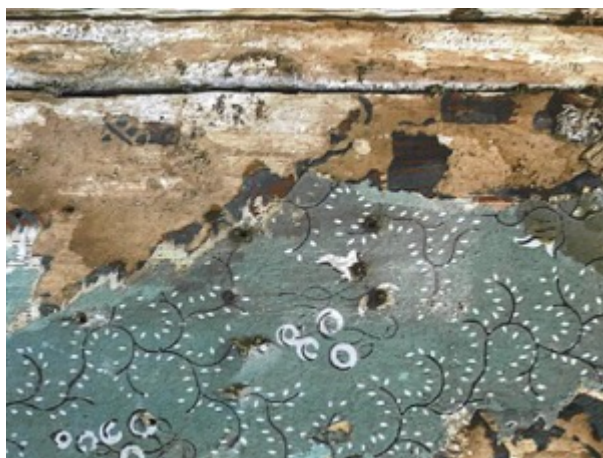
Fig. 1. Detail of wallpaper, showing the upper layer and some of the underlying lower layer.
