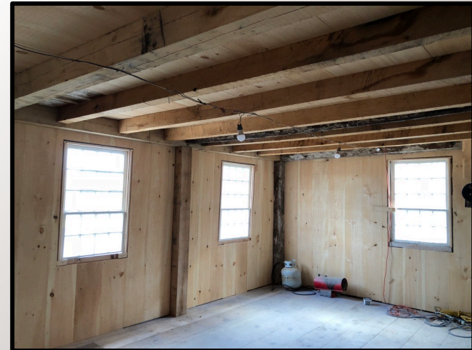
The Keeping Room. Steel posts removed. New beam construction added. Steel brackets for additional stabilization from roof line to plate.
