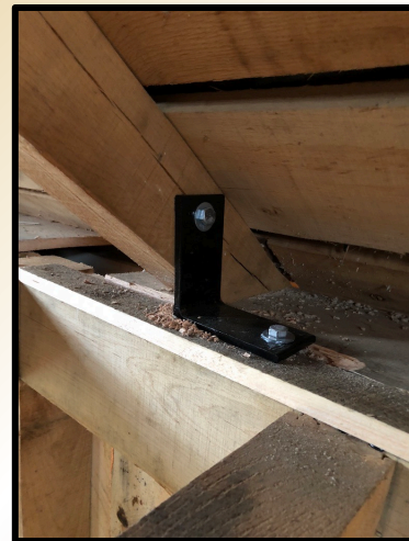
The Keeping Room. Steel posts removed. New beam construction added. Steel brackets for additional stabilization from roof line to plate.
