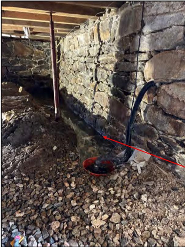
March 25, 2026: additional photos of the French Drain installation. The team had difficulty keeping up with the water while digging two feet.
