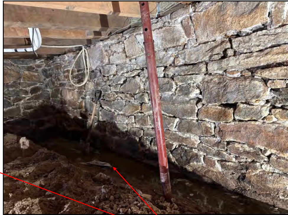
March 25, 2026: additional photos of the French Drain installation. The team had difficulty keeping up with the water while digging two feet.
